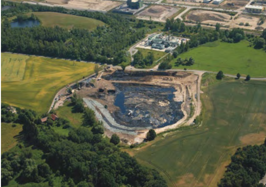
The aerial view shows the extent of the damage caused by the "tar lake".
