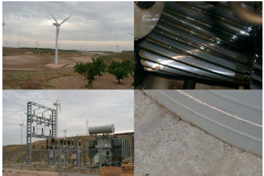
Inspection of wind turbines – San Juan de Bargas Site.
