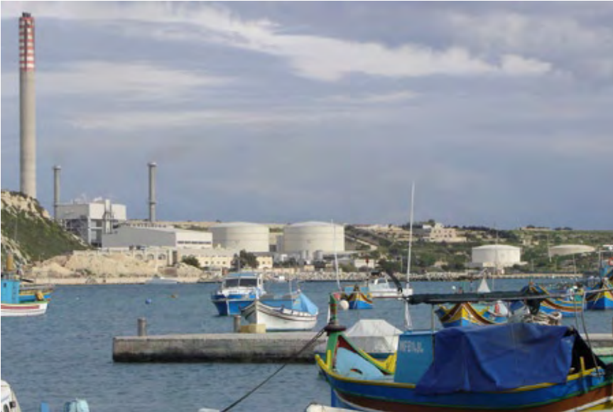
Thermal Power Plant Delimara: mid-term capacity addition by some 260 MW.
