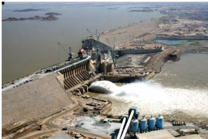
Merowe dam in December 2008.
