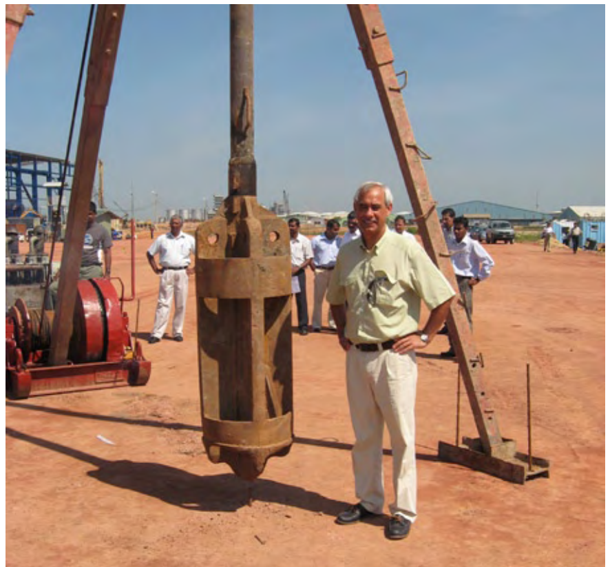
Mr. Ernesto Martínez Telo, GE2 next to pile-driving equipment.
