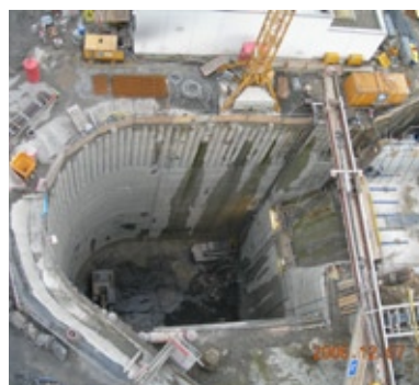
The shaft pit in December 2006.
