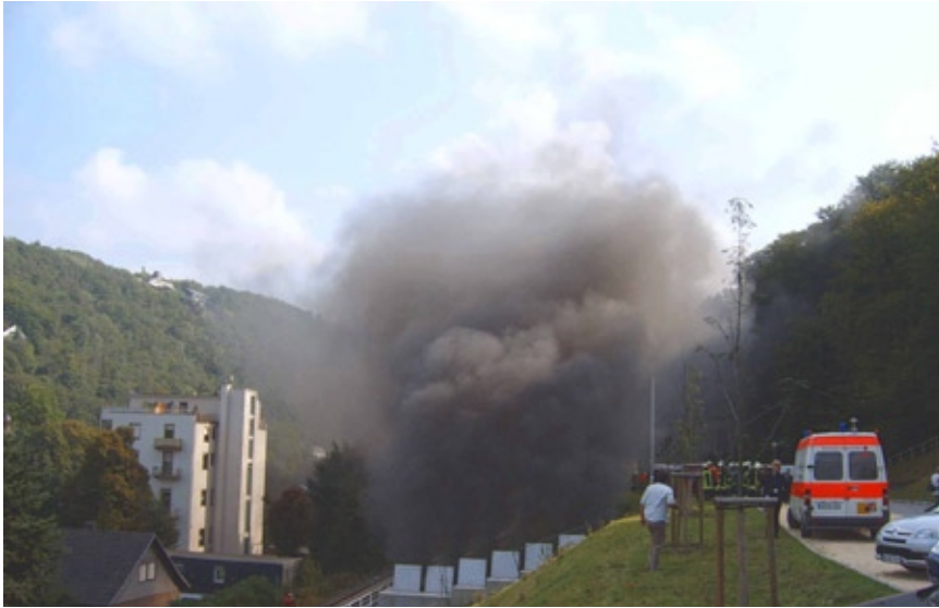
B260 Malberg Tunnel Bad Ems smoke exhaust test.
