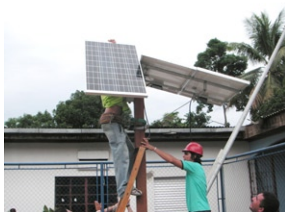
Training of electricians for installation of Solar-Home-Systems in Acre.
