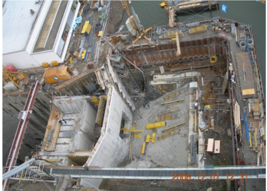
Construction of the outlet works with temporary site enclosure, December 2006.
