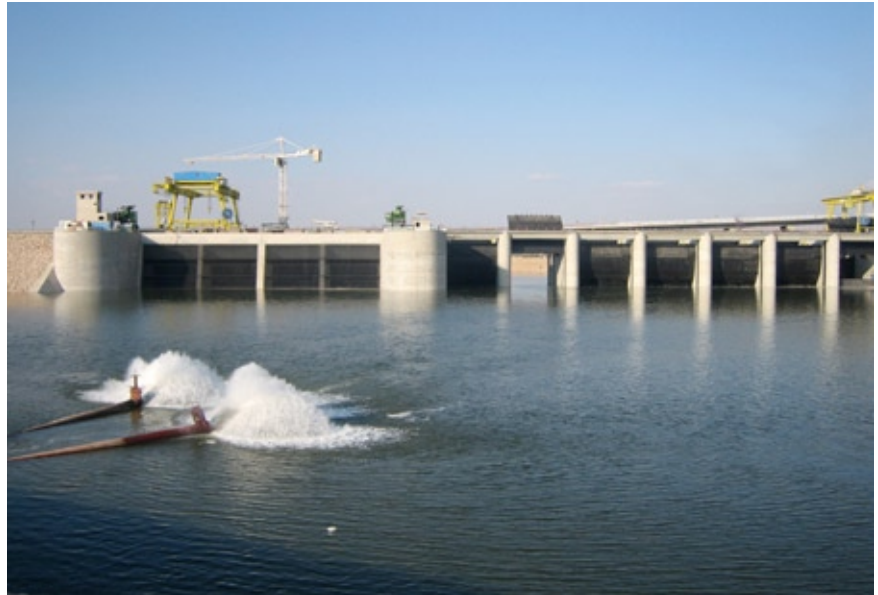
The sluice way with seven bays and radial gates during impounding of the construction pit in December 2006.
