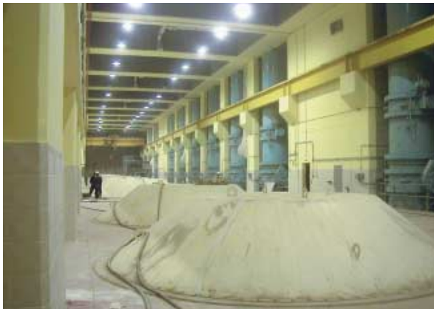
View into the 140 m-long, 14 m-high and 17 m-wide northern pump hall.
