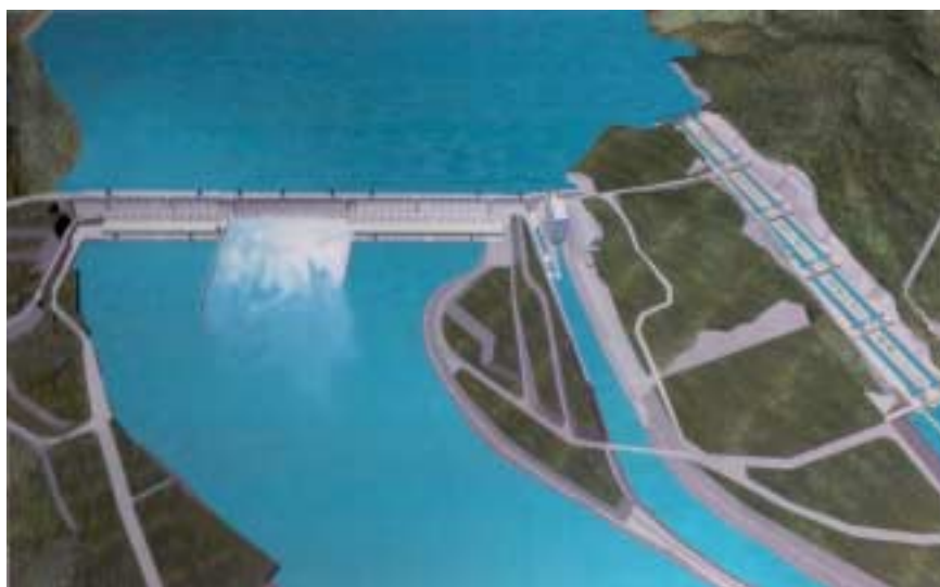
Total view of Three Gorges Project. Structures (from left to right valley flank): flight of locks, shiplift, auxiliary lock for construction period, concrete dam and left-hand powerhouse, spillway, concrete wall and right-hand powerhouse.
