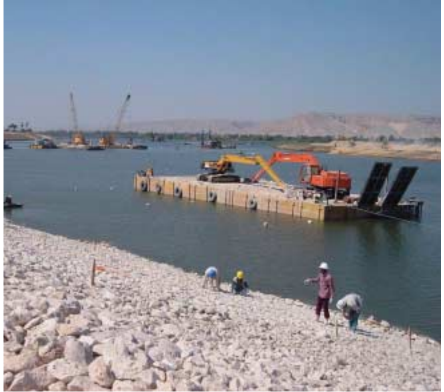
Compaction work in the diversion canal river bed.
