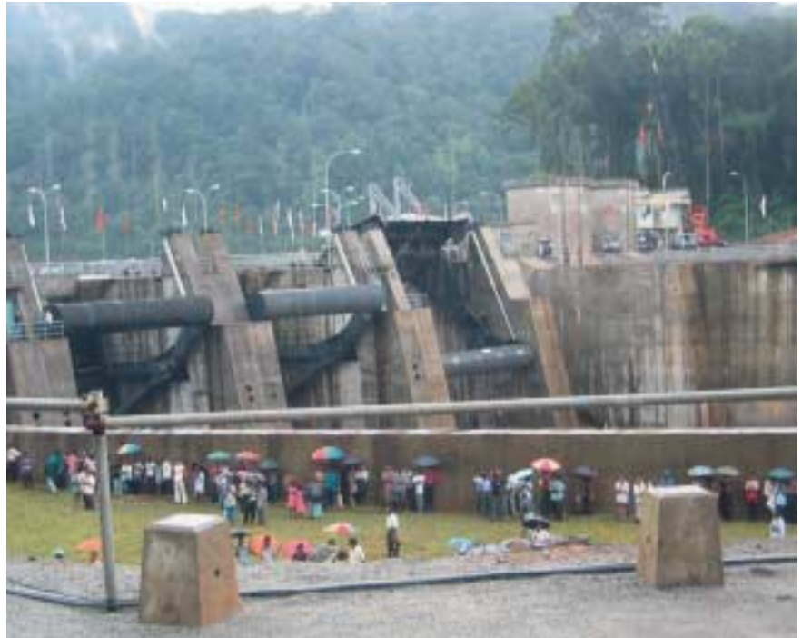
Dam with sectional gates
