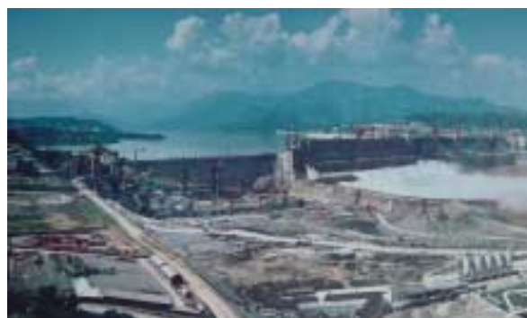
Powerhouse and excavation of dam foundation, right side (from upstream)
