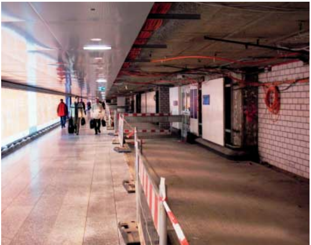
View on the retrofitted junction at 50 % completion.
