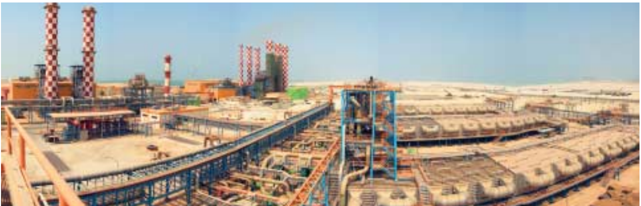
MSF desalination plant Hidd in the Kingdom of Bahrain
